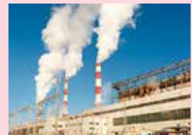
Power Generation Equipment
